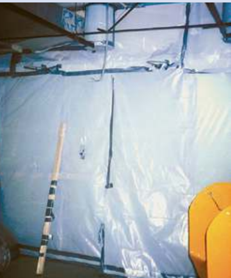
Photo 8: Full containment on large job
